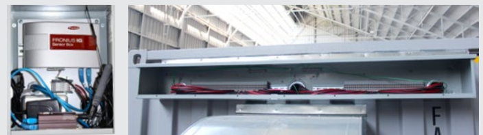
(Top) Inside a finished Anvil Crawler inverter house. (Bottom left) Pre-installed and wired Fronius weather station and monitoring. (Bottom right) Pre-wired inverter DC terminal strip.
